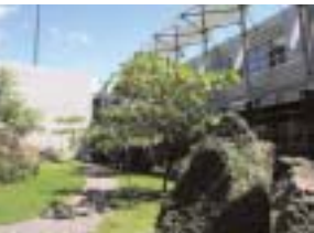
The building design takes advantage of many renewable resources and assets available on the site including sunlight, shade, vegetation, sea breeze, and water.
