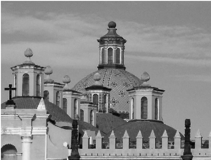
Fig. 5. The Capilla Real of Cholula near Puebla (Mexico) with 49 domes, 23 of which were opened for lighting and ventilating purposes. 6.
