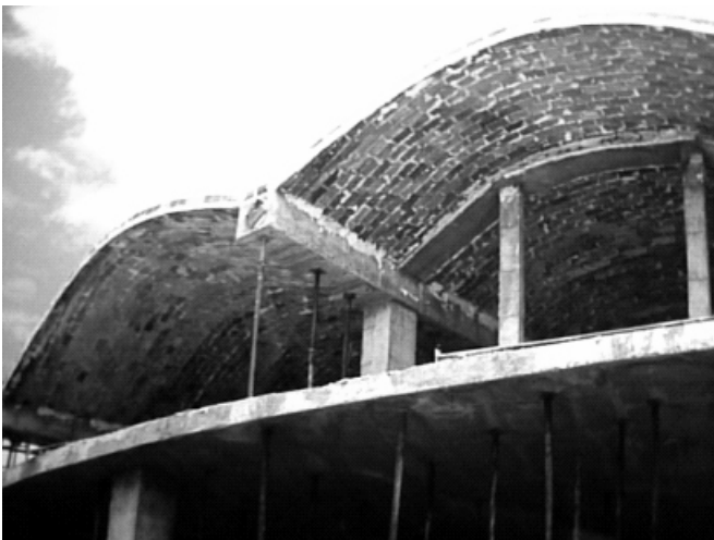
Fig. 24. The central and side vaults of the former house under construction.
