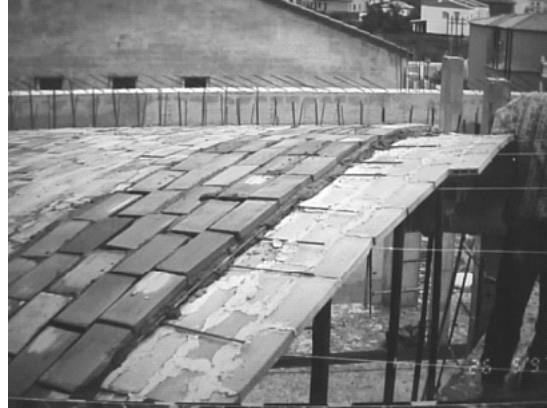
Fig. 22. View of the construction system of the brick vaults.
