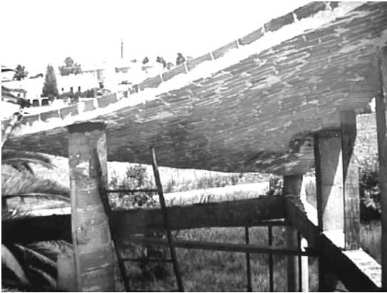
Fig. 21. Interior of a conical brick shell at Calabuig's House in Seville (Spain).
