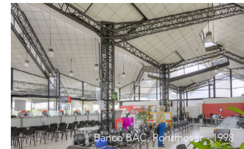
Banco BAC, Rohrmoser - 1998
