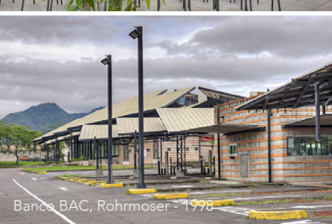
Banco BAC, Rohrmoser - 1998
