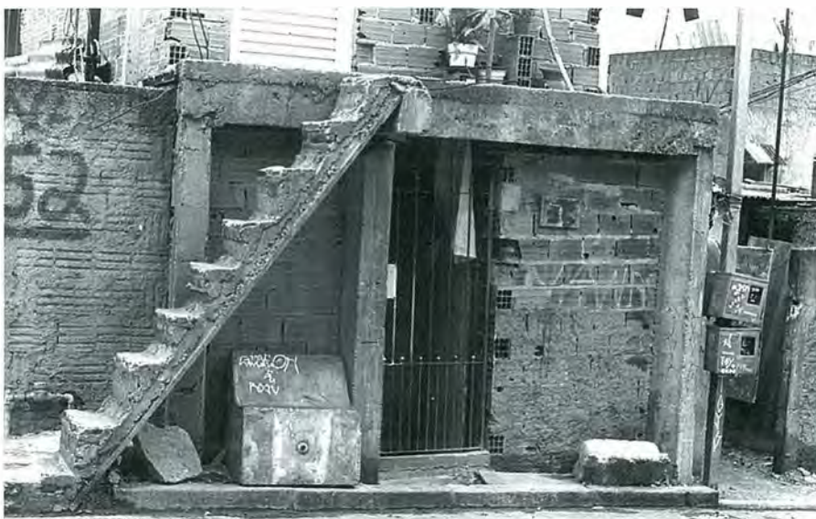
FIGURE 16. Narrow stair that has avoided protruding into the auto-accessible street.
