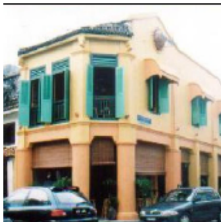
Fig. 16: A shophouse that has undergone adaptive re-use/ Shophouse que ha sido adaptado para reciclarlo.
