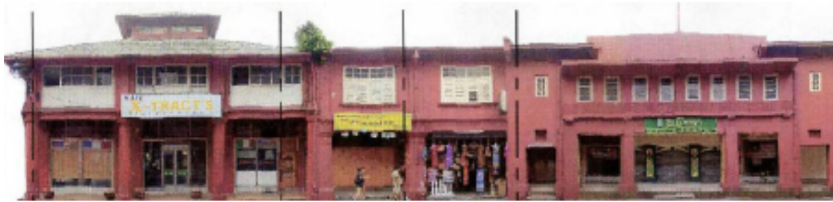
Fig. 13 a: Shophouses along Laksamana Street, Malacca. View from the street / Shophouses en la rivera de la calle Laksamana, en Malasia.
